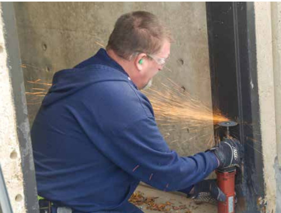
Previous frame rust removal
