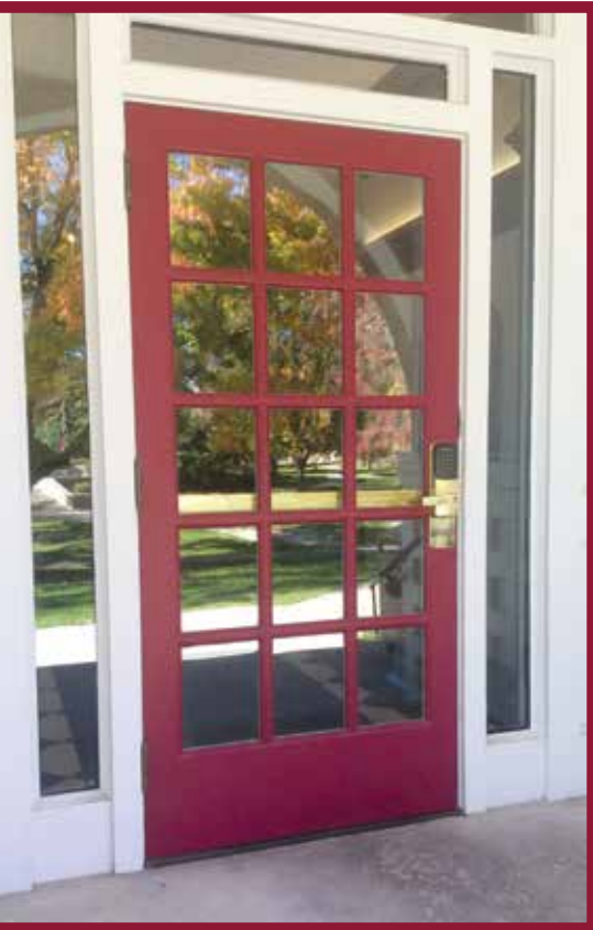
Main entrance to Smith Hall
